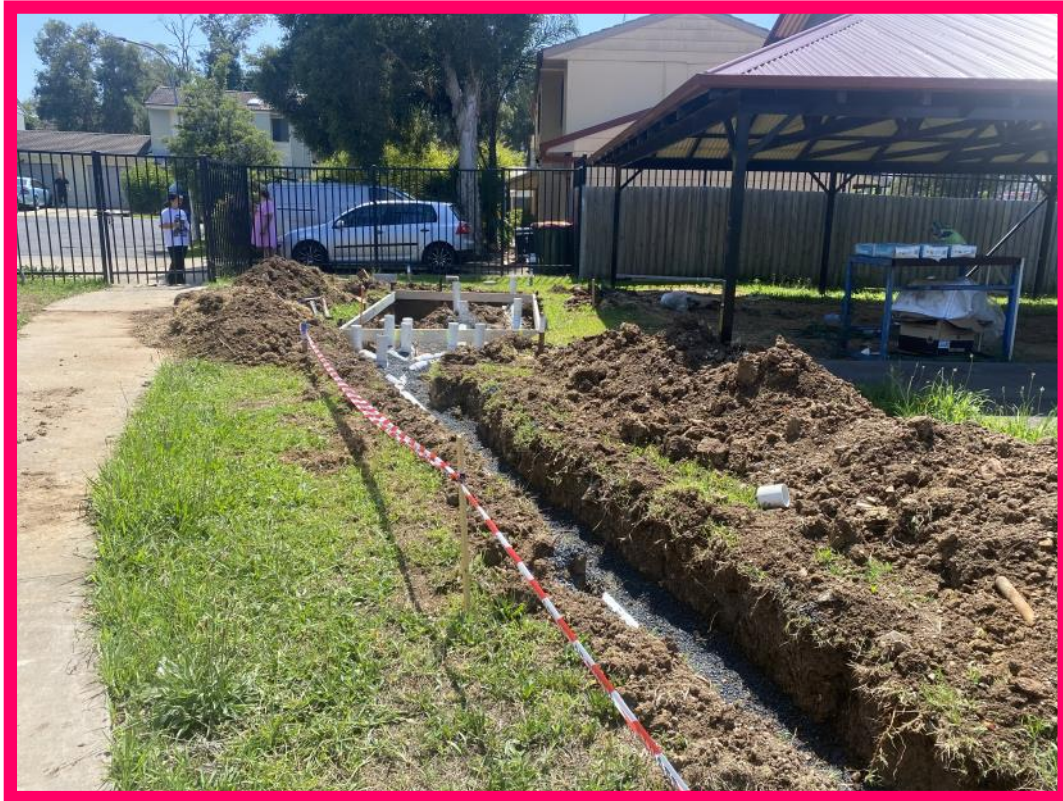
Kwinnie Garden Bathroom Construction November 2023
