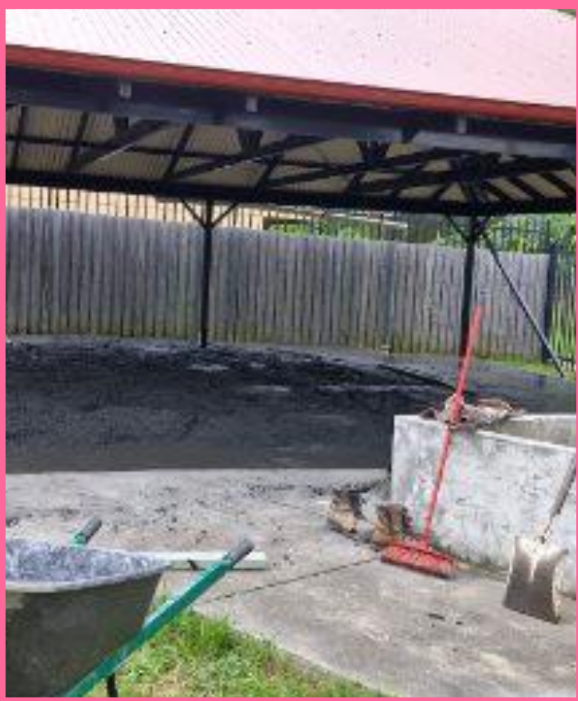
Kwinnie Garden Concrete under Pergola June 2024
